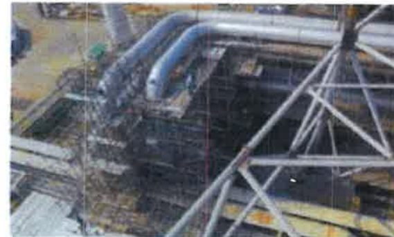
Tie-in 48" Flare Header OLE2-2 Complete
